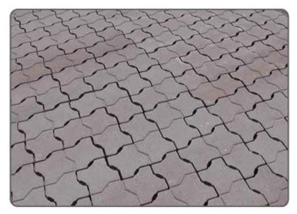
When used as part of Advanced Pavement Technology's exclusive BASS™ method, these pavers allow for natural stormwater drainage and groundwater recharge, making the paved surface ecologically sound and economically smart. In fact, the BASS™ method is an acceptable post-structural Best Management Practice (BMP) used to meet the federal stormwater management requirements. Roads and parking lots created using BASS™ with these permeable pavers qualify for LEED credits and offer vast benefits:
